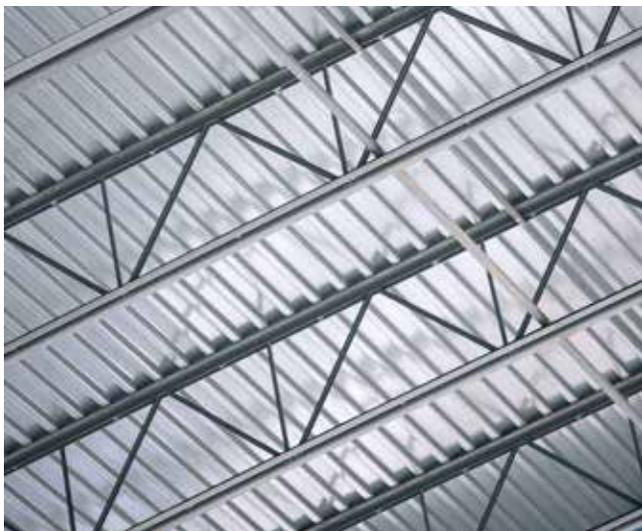
**Steel Joists and Deck**
