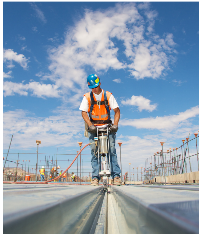
Dek-Lok™ HSL side-lap connection tool operation. The tool is powered by a low-output air compressor.
