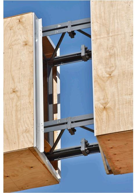
The bridging between the barrel joist trusses connect them all to provide support in more than one direction on the Ford dealership brand wall application.
