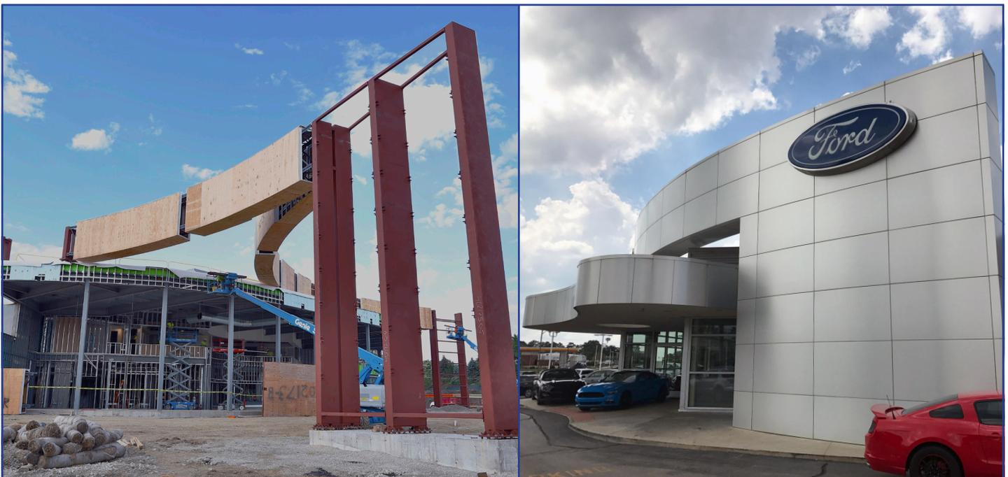
*Barrel joists clad in plywood and connected by custom trusses span the roof of a car dealership under construction (left) and will resemble this previously completed design (right).*
