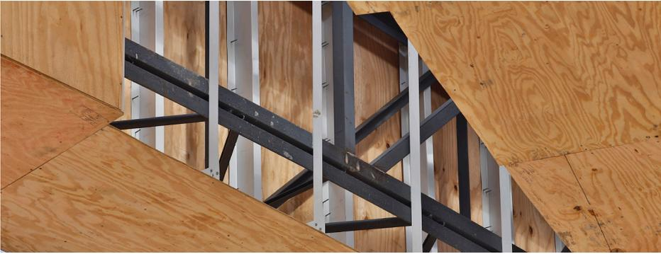
Seen here, a barrel joist is installed on its side and supported by webbing to create a box truss that can handle both downward gravity loads and sideways wind loads.
