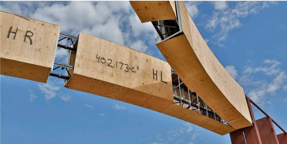
New Millennium delivered the barrel joist box trusses to the customer fully assembled, along with detailed field drawings to aid in proper installation to speed erection and ensure correct and safe on-site construction.
