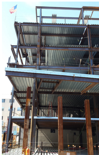
A 13-inch deep Versa-Floor™ Deep-Dek® Composite system addressed strength, openness, and vibration control challenges.
