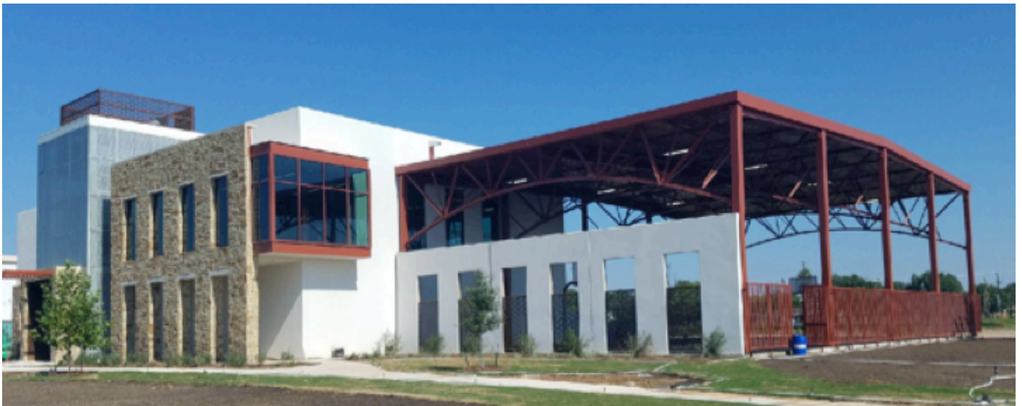
The exposed joist framing system for the Harvey E. Najim Family YMCA "Air-nasium" — a 6,500 sq. ft. outdoor gym — features joist girders with curved bottom chords to meet both structural and aesthetic requirements of the project.
