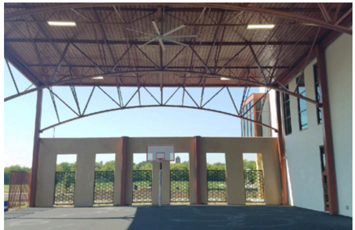
New Millennium designed an aesthetically pleasing curved bottom chord joist girder system with square HSS bracing that the architect preferred to retain the aesthetic goal of the project while keeping costs down.
