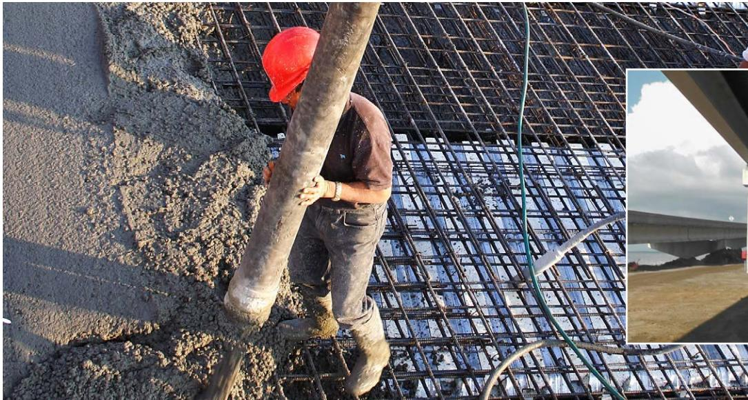
New Millennium's Bridge-Dek® and Rhino-Dek® stay-in-place steel form systems allow project owners to reduce costs by 20-25%, compared to wood forms.
