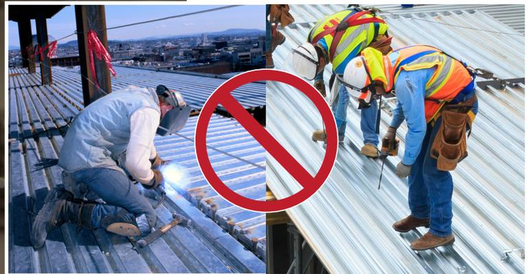
*Labor intensive and back-breaking... traditional methods of installation may soon give way to the use of automated tools for steel deck side lapping and support fastening.*
