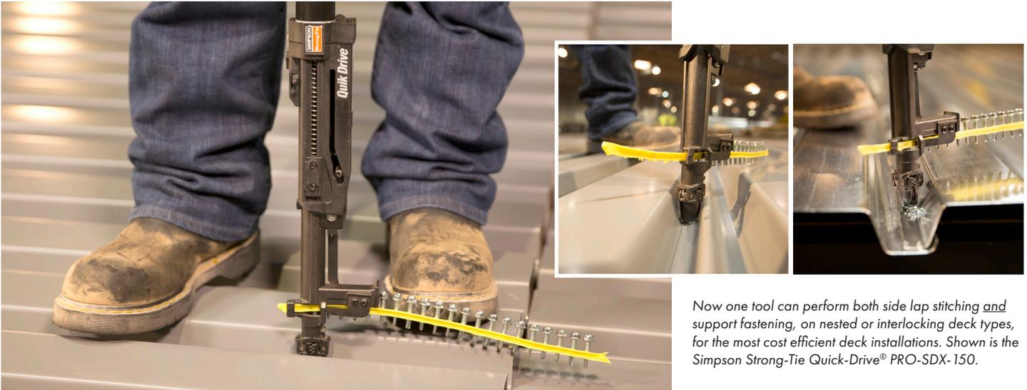
Now one tool can perform both side lap stitching and support fastening, on nested or interlocking deck types, for the most cost efficient deck installations. Shown is the Simpson Strong-Tie Quick-Drive® PRO-SDX-150.
