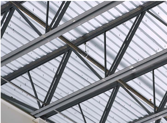
The open-web design of a steel joist provides strength and versatility.
