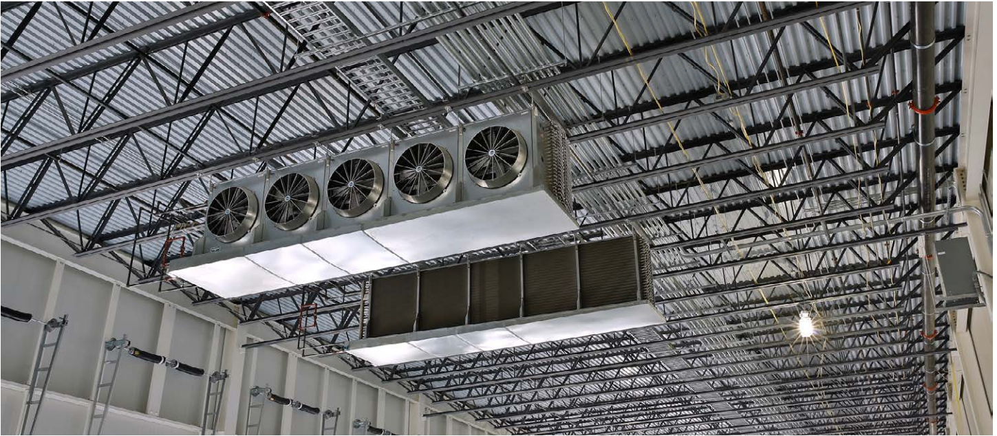
Single-piece joists can span up to 120' and with a bolted splice assembled in the field can span up to 240'. As a roof or floor system, they are capable of efficiently supporting nearly any demand imposed upon them.
