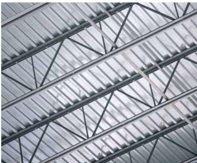
**Steel Joists and Deck**
