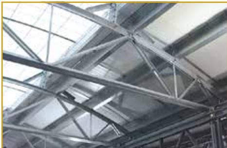
Flex-Joist™ tension-controlled steel joist design is ideally suited to electronic monitoring of deflection and/or strain for early warning of high loads, if desired. This can allow time for building evacuation, load removal, and/or shoring to prevent collapse. Although electronic monitoring is not provided by NMBS, we can help coordinate requirements with your electronic monitoring supplier.
